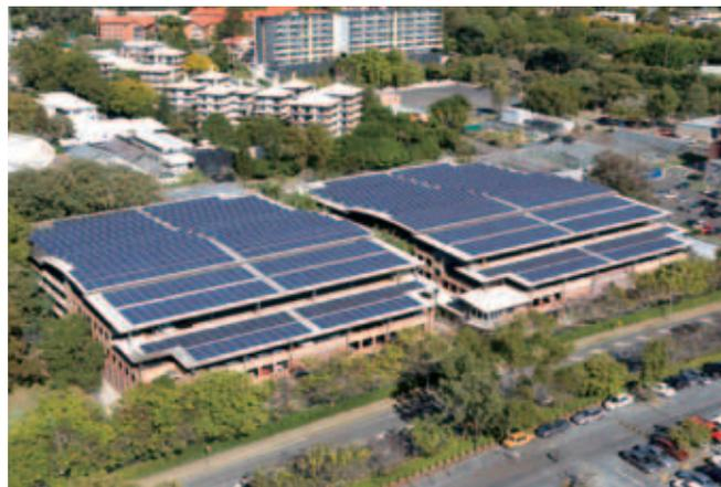
The inclusion of a 200kW battery bank, connected to a 400kWp section of the installation, allows research into solar power capture techniques during the day and feeding it into the grid at night and other peak times.
